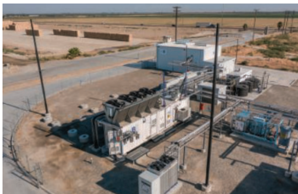
At SoHyCal's hydrogen plant near Fresno, California, biogas from manure powers fuel cells, which supply green electricity to electrolyzers.
